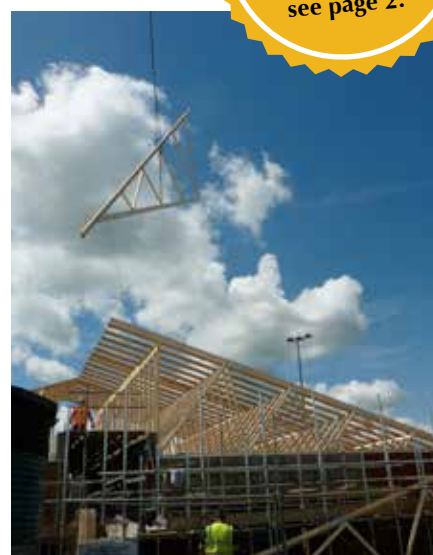
... and the roof's going on!
