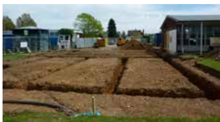
The footings are dug
