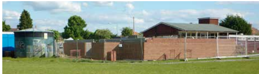
... the walls are up
